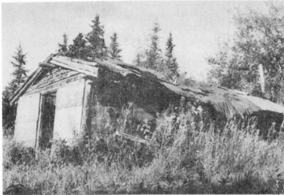
Plate 70 — Hogan Hill cabin built circa 1927. Cabin is on the highway right-of-way. (BLM photo.)
