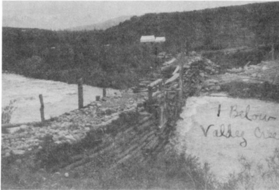
Plate 7 — Dam on No. 1 below Discovery for sawmill race, 1905. (From Crary-Henderson Collection, Anchorage Historical and Fine Arts Museum.)
