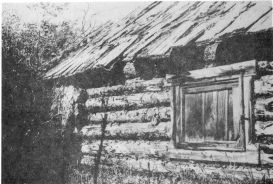
Plate 61 — Repair shop, northwest corner, in 1977 just before it was destroyed. (BLM photo.)
