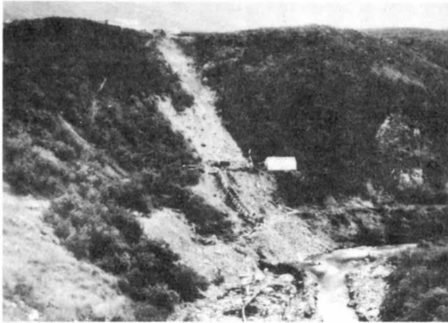
Plate 15 – Monahan Tunnel into the bottom of the Tammany channel, 1917. (From Moffit 1912: Plate IX.)
