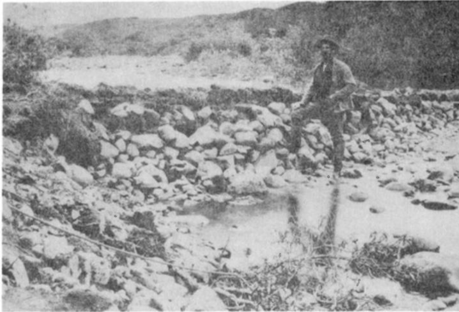
Plate 9 – Dam on upper tributary of Valdez Creek. Man in photo is Lou Powless. (From Crary-Henderson Collection, Anchorage Historical and Fine Arts Museum.)
