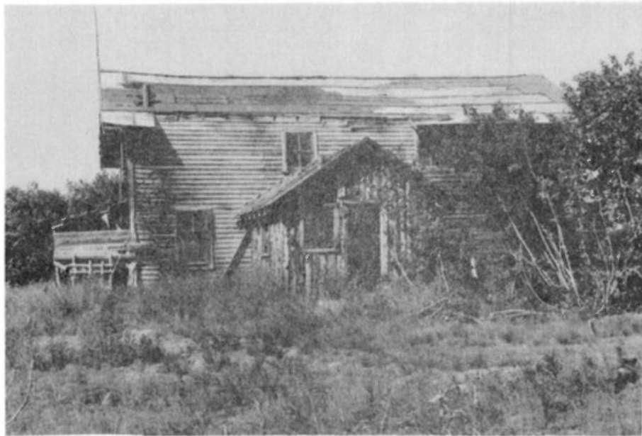
Plate 54 – Denali bunkhouse, east side, 1977 just before it was destroyed. (BLM photo.)
