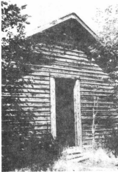
Plate 56 – North building, south end, in 1977 just before it was destroyed. (BLM photo.)
