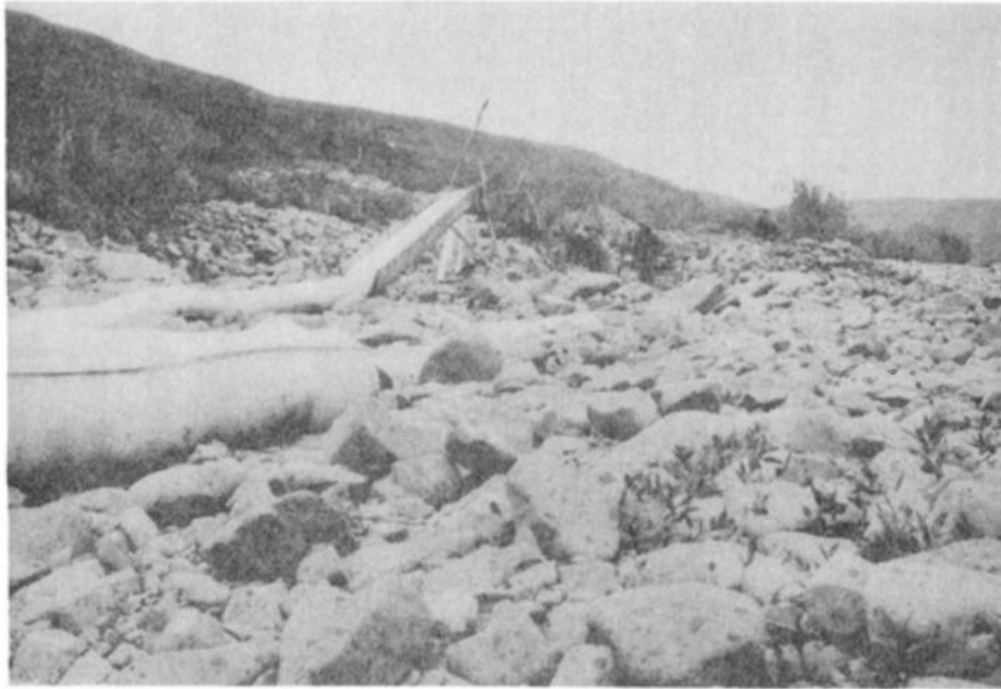
Plate 10 – Canvas pipe and sluice box at placer site below the dam. (From Crary-Henderson Collection, Anchorage Historical and Fine Arts Museum.)
