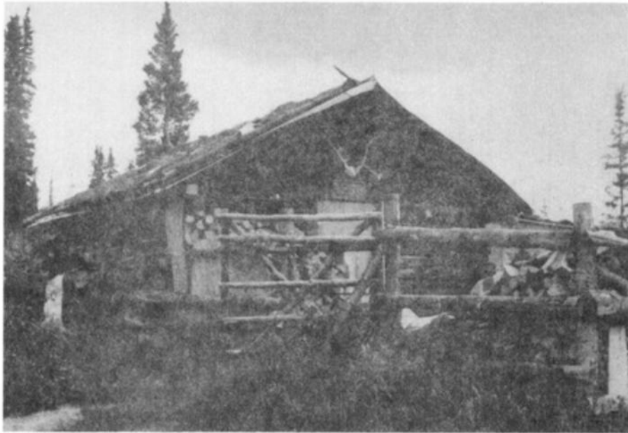
Plate 80 – Thirty-Mile Shelter cabin built in the 1920's. (BLM photo.)
