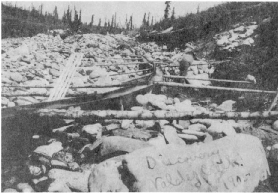
Plate 5 — Shovelling pay dirt into sluice box on Discovery Claim, 1905. (From Crary-Henderson Collection, Anchorage Historical and Fine Arts Museum.)
