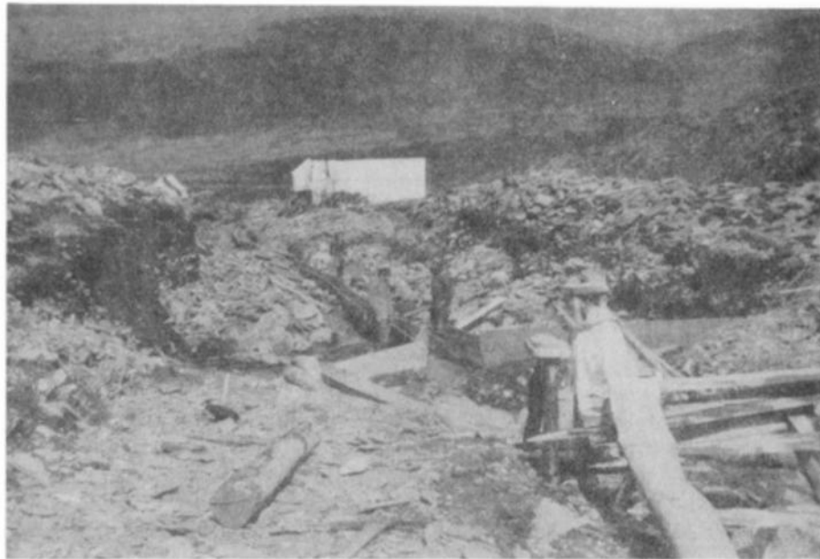
Plate 12 – Sluice box on Lucky Gulch for hydraulic operation. (From Crary-Henderson Collection, Anchorage Historical and Fine Arts Museum.)
