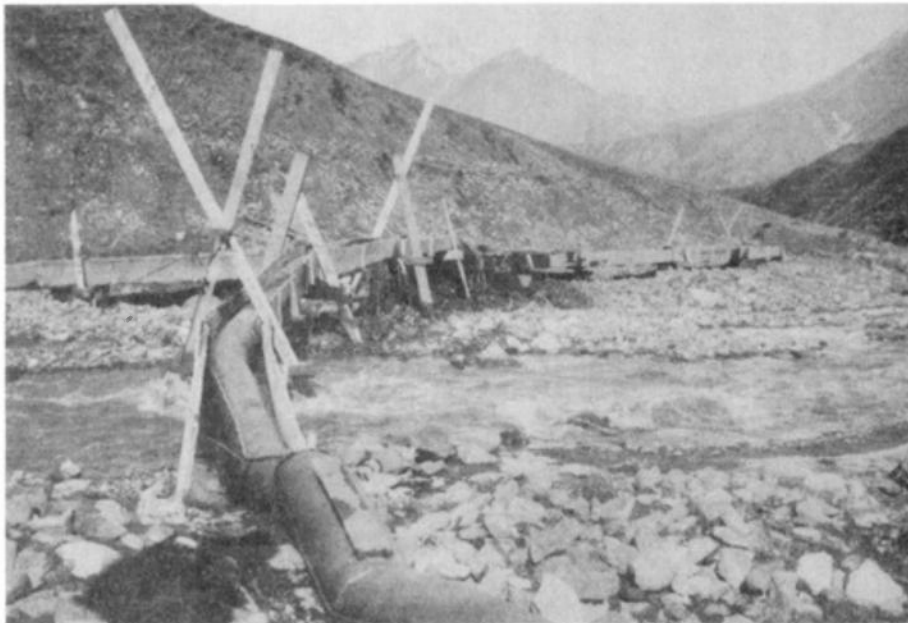
Plate 8 — Canvas pipe and flume on Timberline Creek. (From Crary-Henderson Collection, Anchorage Historical and Fine Arts Museum.)
