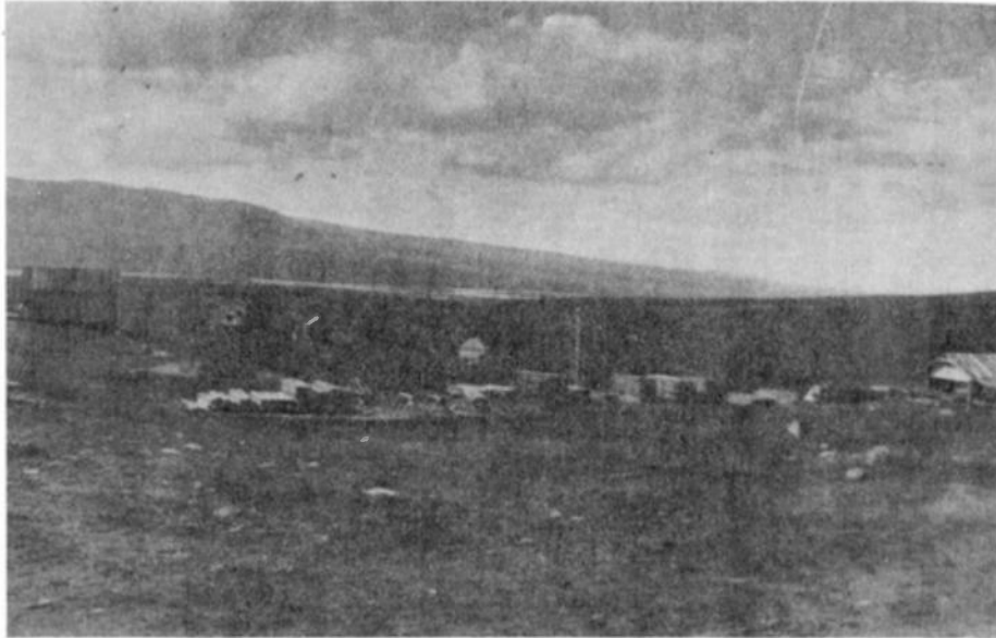
Plate 17 – Store, sawmill and tent cabins at Denali, circa 1918. (From A. B. Smith, Big Delta.)
